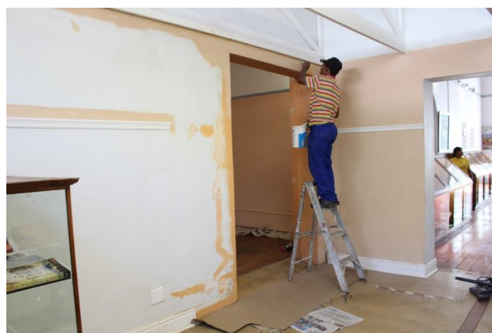
The new doorway to the Rock Art Room
